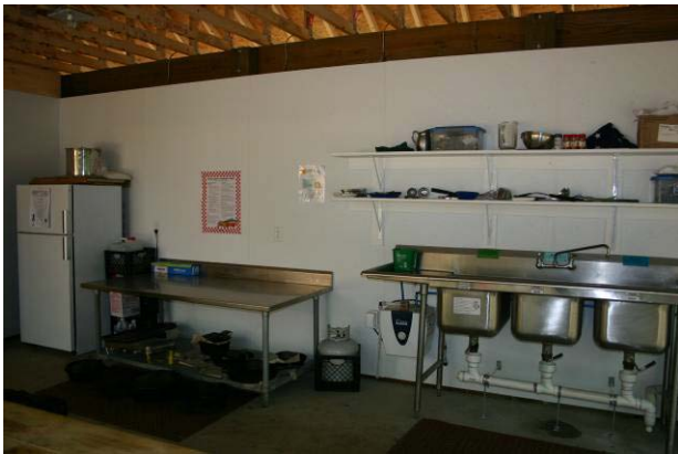
The kitchen facilities in the Cooking Merit Badge pavilion are complete with running water and refrigeration.
