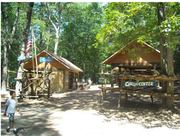
The newly-completed Campcraft Center
